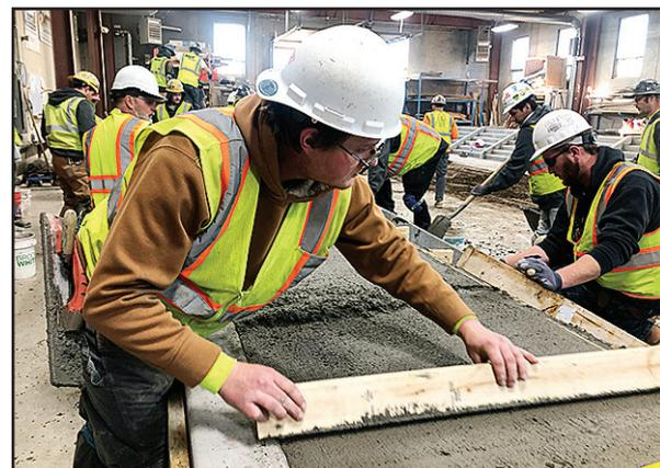
*Photo above, right:* Third-year apprentice Ben Franzen, St. Cloud, striking off the 3-foot landing elevation with a rod board.
